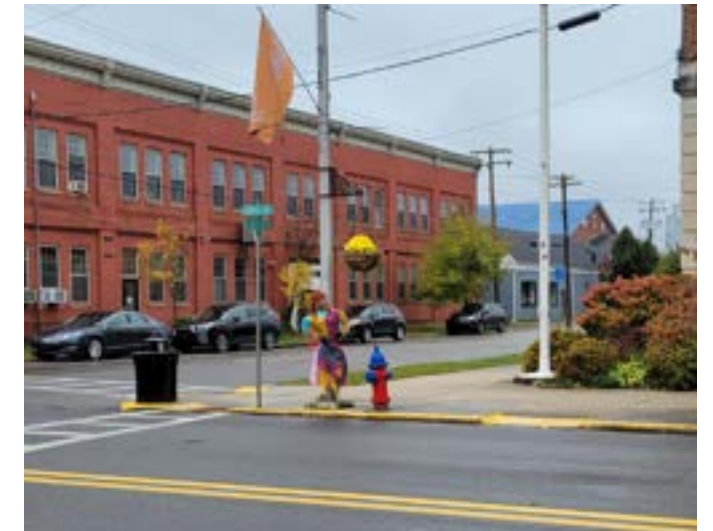
Existing crosswalk and ADA curb cuts with ramps at the intersection of Davis Avenue and 4th Street.
