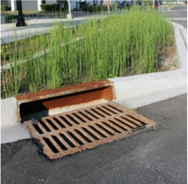
Low vegetation within bumpouts for stormwater filtration and clear sight lines.
