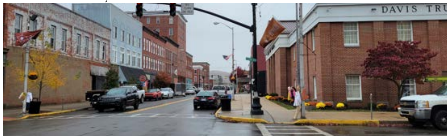
Existing intersection at 3rd Street and Davis Avenue
