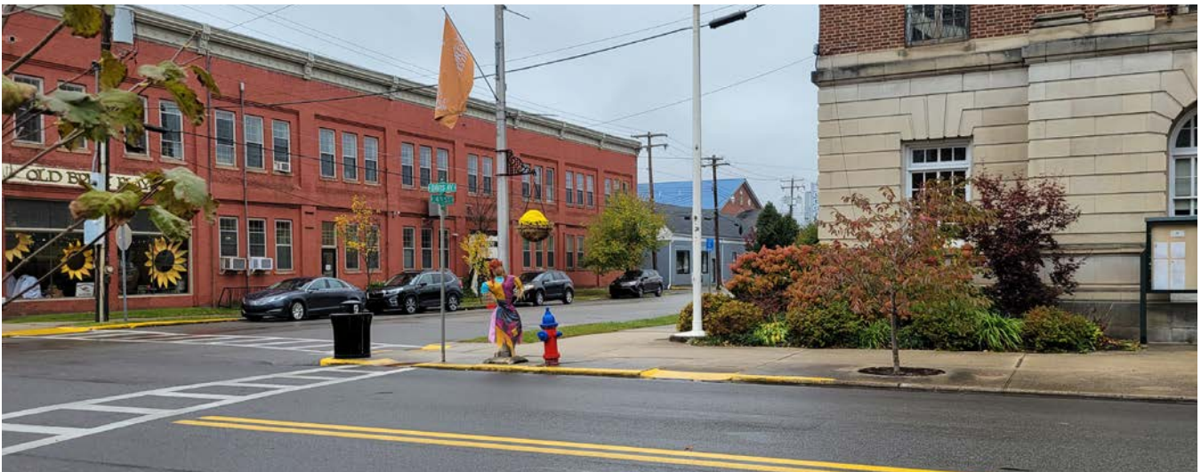
Existing crosswalk and ADA curb cuts with ramps at the intersection of Davis Avenue and 4th Street.
