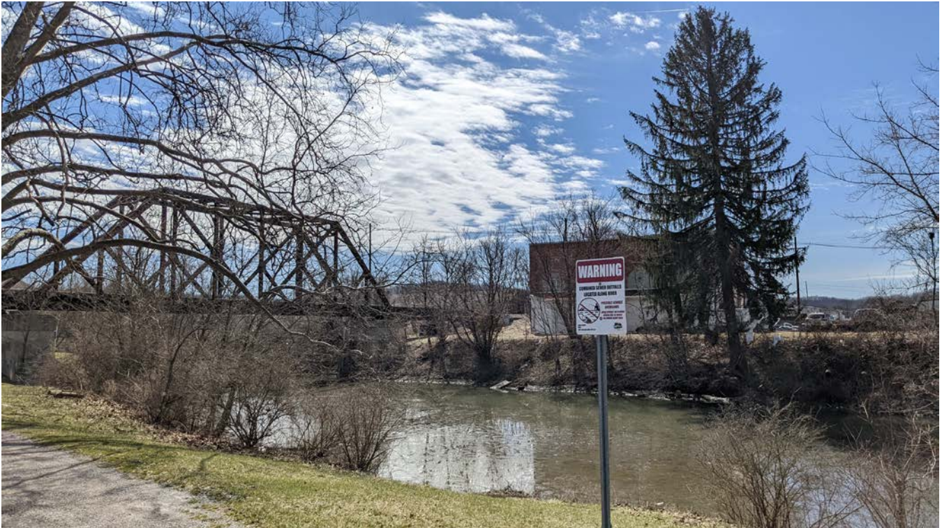
Existing rail trestle bridge crossing the Tygart Valley River near the rail depot to be considered for pedestrian connection over the river towards downtown utilizing a cantilevered trail extension.
