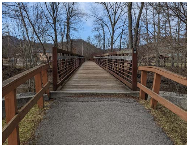
Pedestrian bridge between River Bend and Glendale Parks provided a connection over the river that can be replicated in other areas of the trail system.
